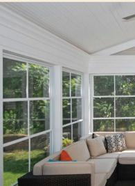
products are constructed with durable aluminum frames that hold screen and vinyl glazed panels in place. Lightweight...
